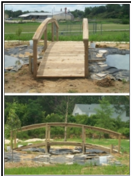
Footbridge and Pond Construction
