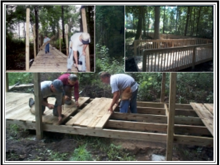
Will Arthur, Mike Branyon, Jerry Blue, and Danny Driggers during boardwalk construction.
